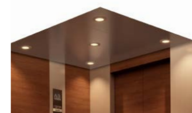
Ceiling: L210S LED downlights (yellow-orange)
